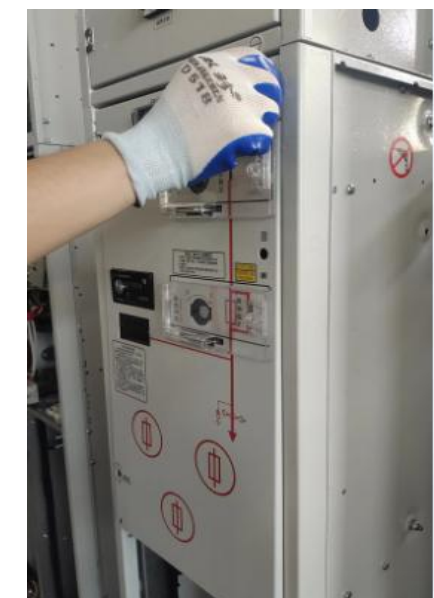
2.松开螺丝,打开熔断器面板
